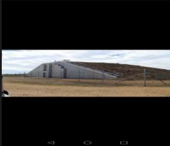
Portable Surface Magazine Lined, ventilated — approved for initiating devices
